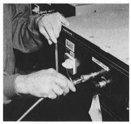
13. Reset the two buttons under the front panel of the compressor. (One button is slightly above and the other slightly below the centre of the hole.)
