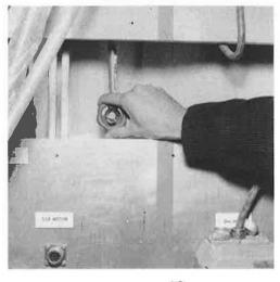
3. Reset the two buttons under the front panel of the compressor. (One button is slightly above and the other slightly below the centre of the hole.)
