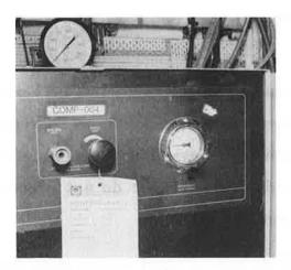
4. Open the black gas valve on the compressor front panel and lower the pressure to ca. 21 bar. If the compressor cuts-out again: lower the pressure by 0.5 bar, close the black gas valve and start again from item 2.
