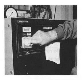
2. Check the water supply line and ensure that the water taps are fully open.
