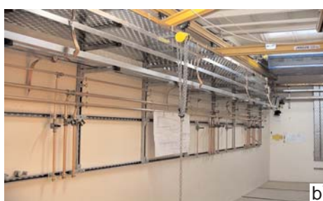
Figure 7 - Views of I22 during installation a) Transfer line showing Experimental hutch, b) internal detail of Optics hutch showing tray work and services supply pipes, c) Overview of I22 area, optics hutch to right and experimental hutch to left. Installation of the steel-work to support the user and control cabins is underway in the middle d) View showing the Controls and Instrumentation Area (CIA) areas and in background the User cabin..
