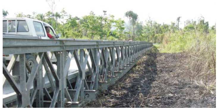
Floods can transport a huge amount of sediment into oceans and onto reefs. At this bridge in PNG the whole river channel was filled up with sediment over a distance of 20 km. The river channel disappeared altogether within 3 - 5 years. This bridge worth a million kina became redundant and was dismantled.
