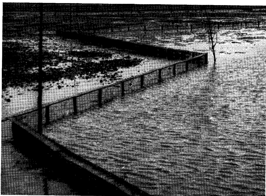
A low fence with projecting horizontal top to prevent access by crabs.
