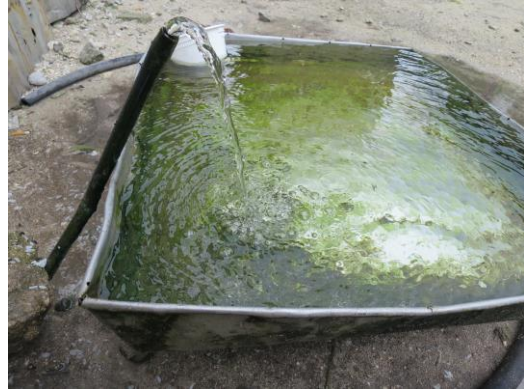
Open pipe, with continuous flow at ground level.
