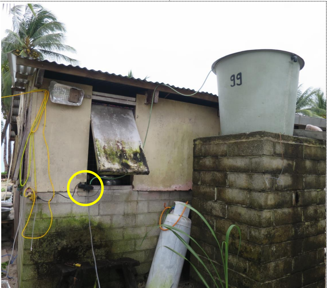
Booster pump at house lifting water into 500 L header tank.
