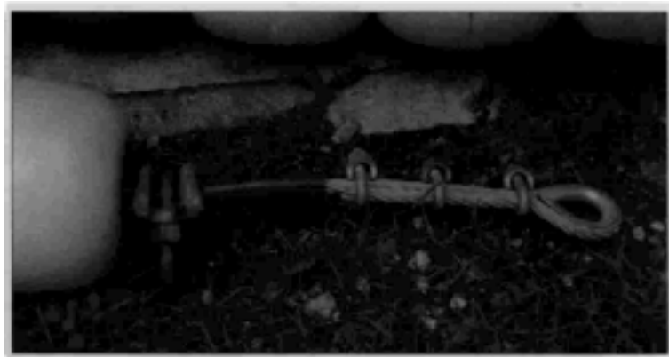
Figure 27: Eye splice formed using cable clamps at end of wire cable
