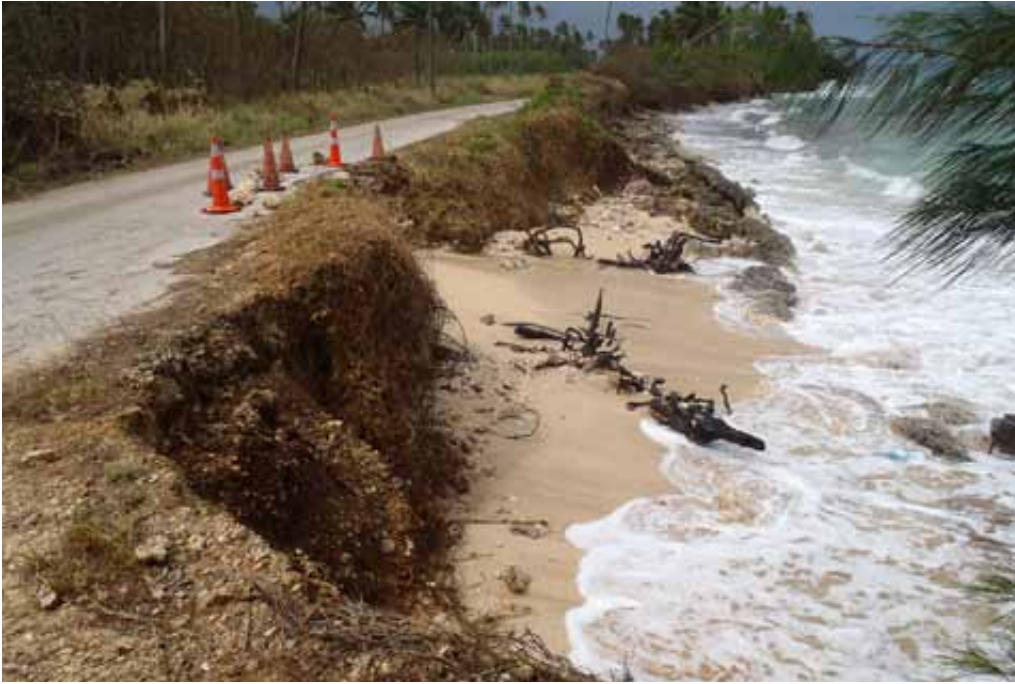
Figure 13. Road in Lifuka affected by coastal erosion following TC Jasmine
