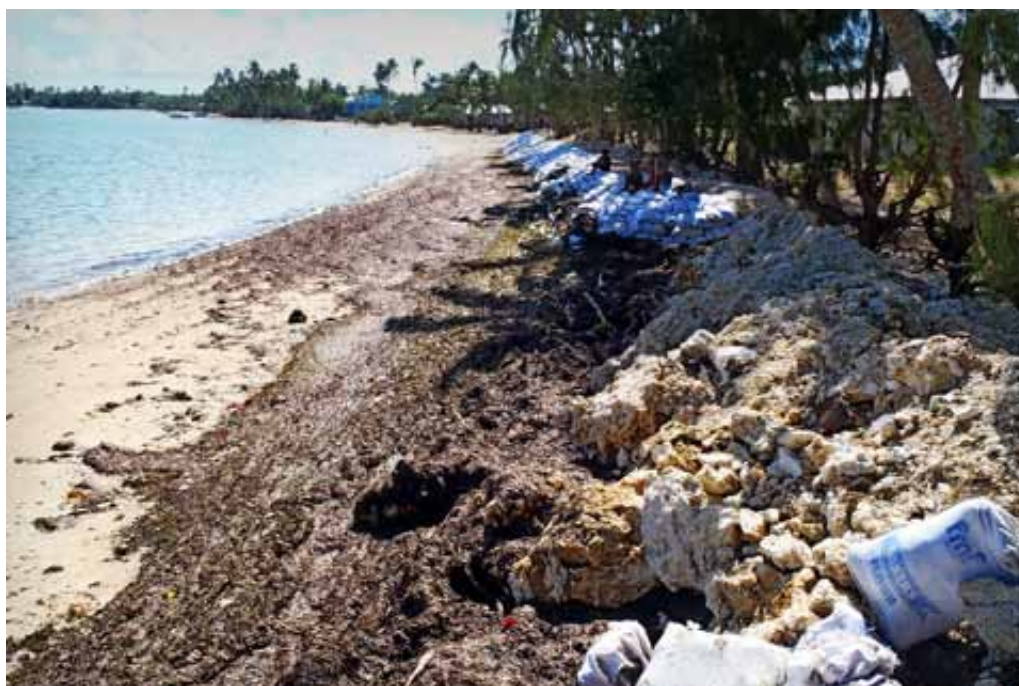
Figure 11. Sea wall in front of Lifuka Hospital
