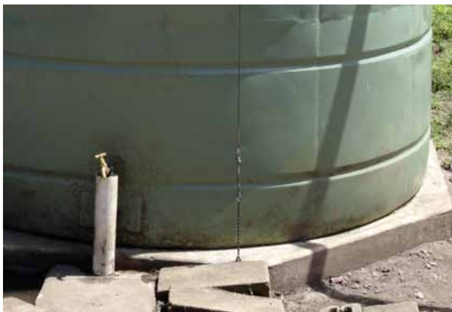
Figure 17. External tap on a plastic tank
