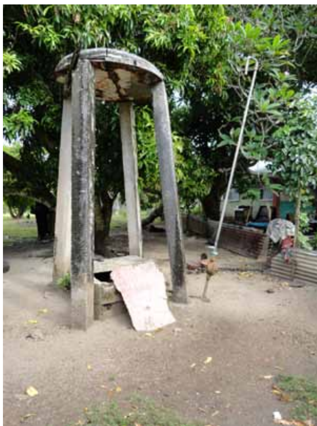
Figure 60. Domestic well in Hihifo, Lifuka, in use, where the manual pump and header tank have been replaced with a bucket
