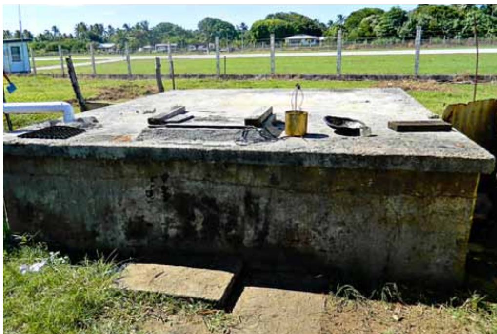
Figure 2. Connected cement cistern
