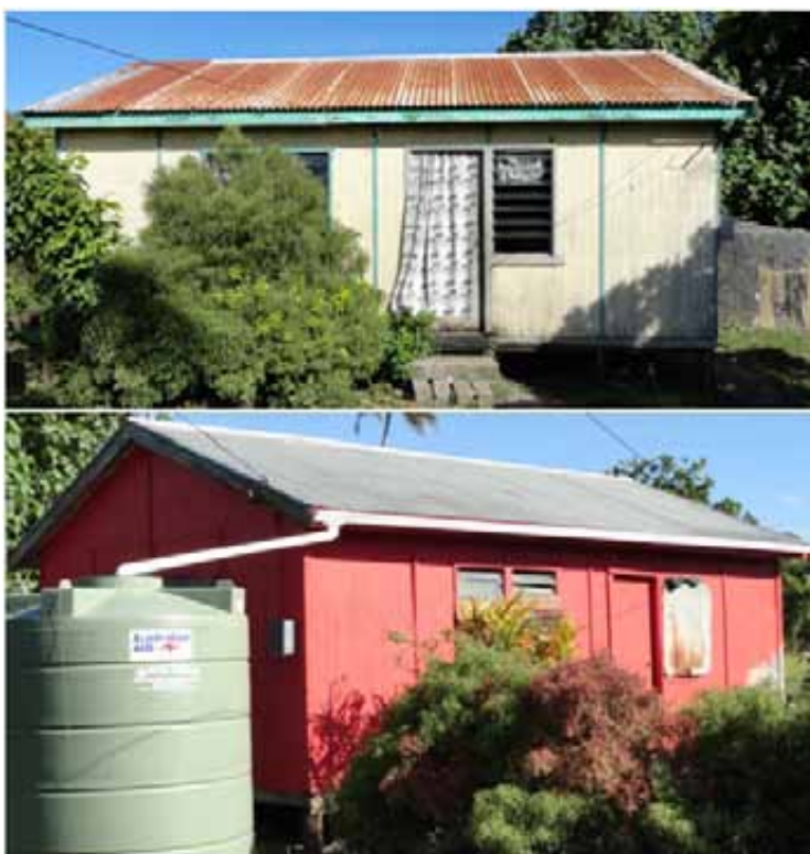
Figure 2. A rusted roof (top) and one in good condition
