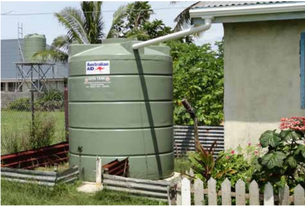
Figure 4. Connected plastic tank
