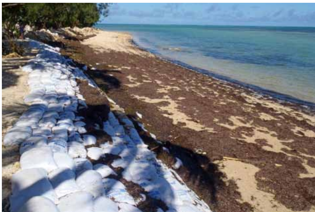
Figure 12. Sea wall in front of Lifuka Hospital
