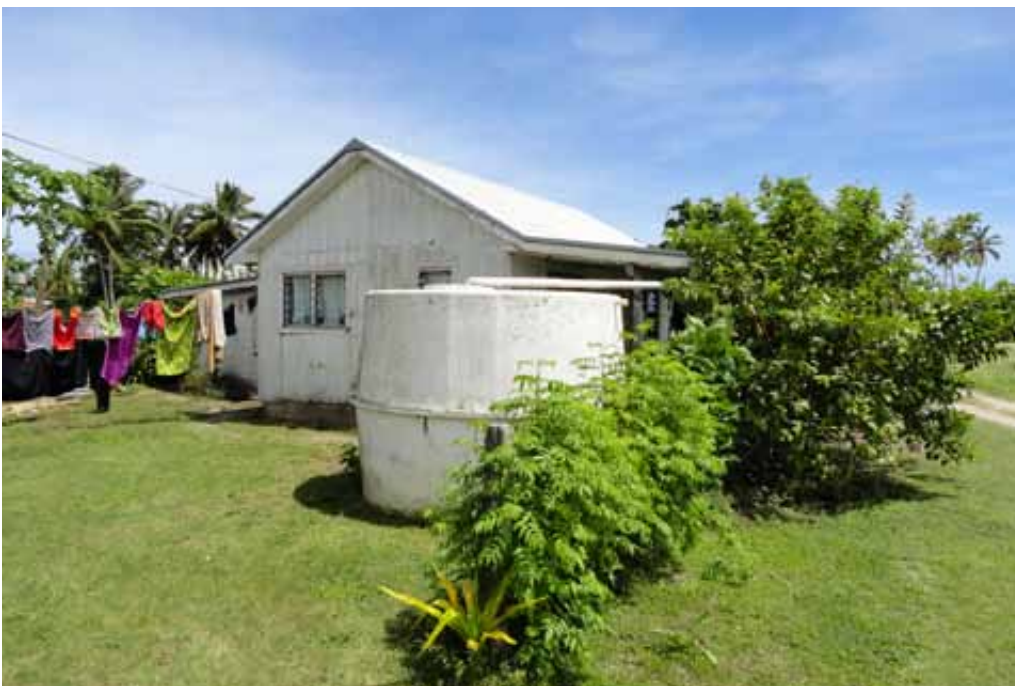
Figure 5. Connected fibreglass tank
