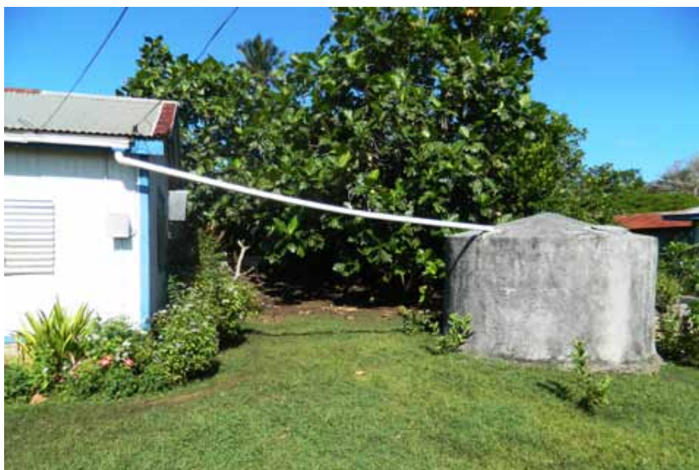
Figure 3. Connected cement tank
