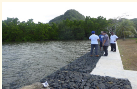
Completed gabion seawall
