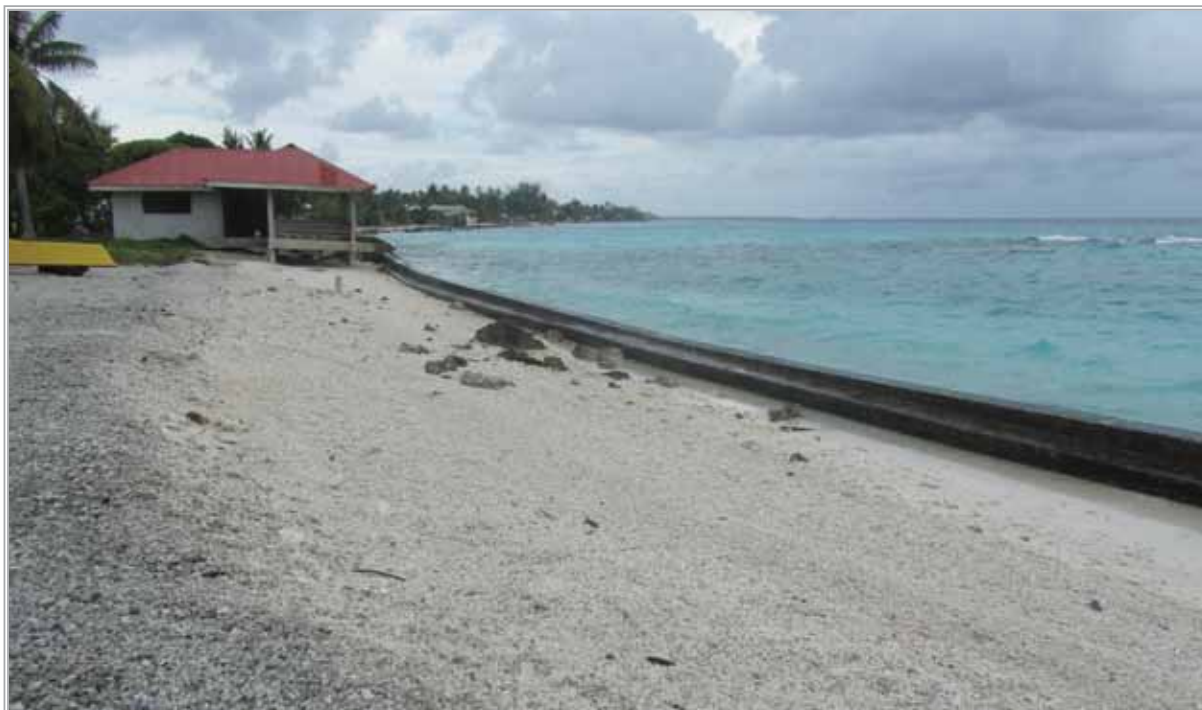
Figure 6: A bulkhead on the lagoon side of Avatoru, with beach erosion still unprevented. Image: Anna Rios Wilks (Dec, 2012).
