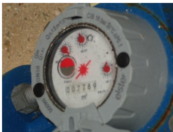
Figure 20: FFM at gallery 12 showing 7789.994 m 3 several minutes after photo at Figure 17 was taken, indicating that there was no water flow and suggesting that the pump may not be working, even though the motor was on.
