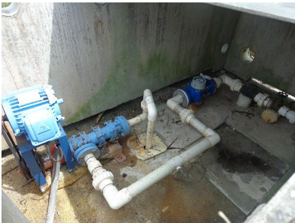
Figure A4.6: Typical pipe work set up in the gallery pump house characterised by numerous bending and connections and causing highly turbulent flow. These will need to be modified to allow more pipe length before the FFM installation to allow more laminar flow and to permit the accurate estimation of discharge flow.
