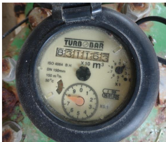
Figure 3: FFM at the WTP outlet in Bonriki reading 8311631.77 m 3 .
