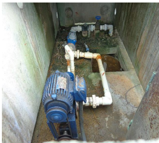
Figure 6: Typical layout in a gallery pump house, comprising the pump motor, FFM, non-return valve and a gate valve. The numerous pipe bending and connections are likely to cause turbulent flow and generate erroneous flow readings.
