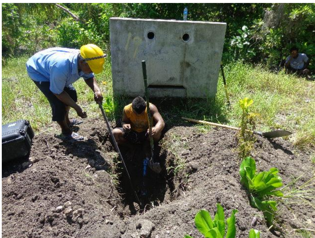
Figure A4.8: PUB staff and a casual labourer digging and exposing the gallery 19 pipe.
