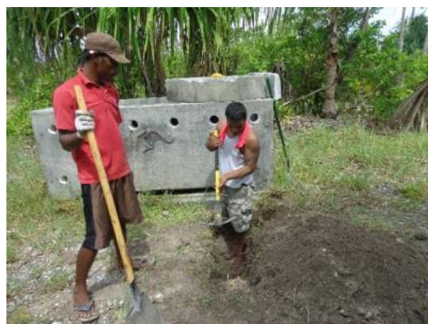
Figure 10: Excavation team digging down to the drainage line for gallery 16.
