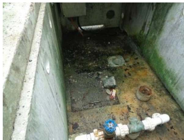
Figure 9: Gallery 2 showing no pump due to previous electrical failure.
