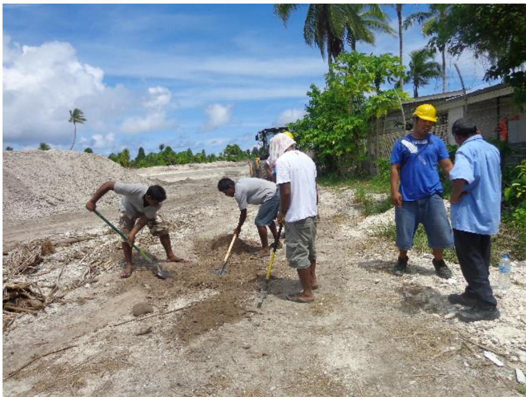
Figure A4.1: Survey team digging to locate the transmission pipe 10 m away from the Bonriki WTP master meter.
