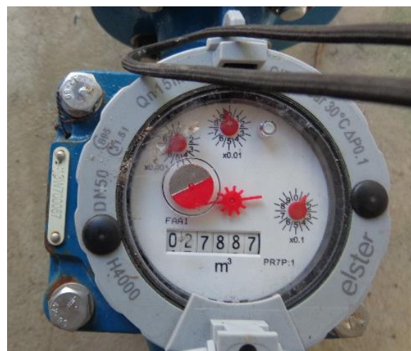
Figure 4: FFM at gallery 13 pump house reading 27887.096 m 3 .
