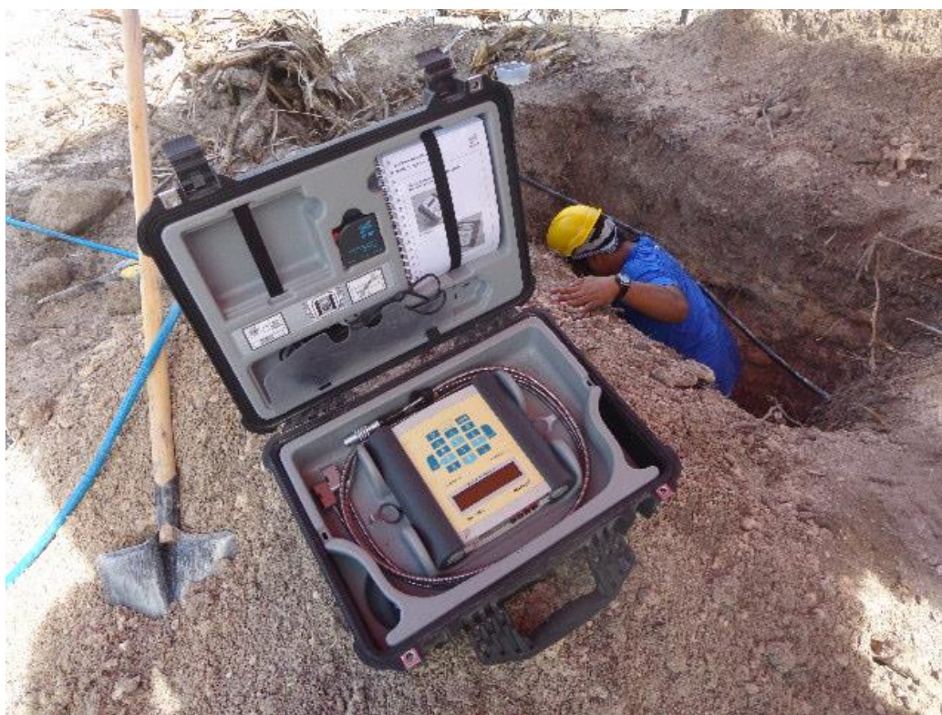
Figure A4.2: PUB staff cleaning the Bonriki transmission pipe before installing the UFM.
