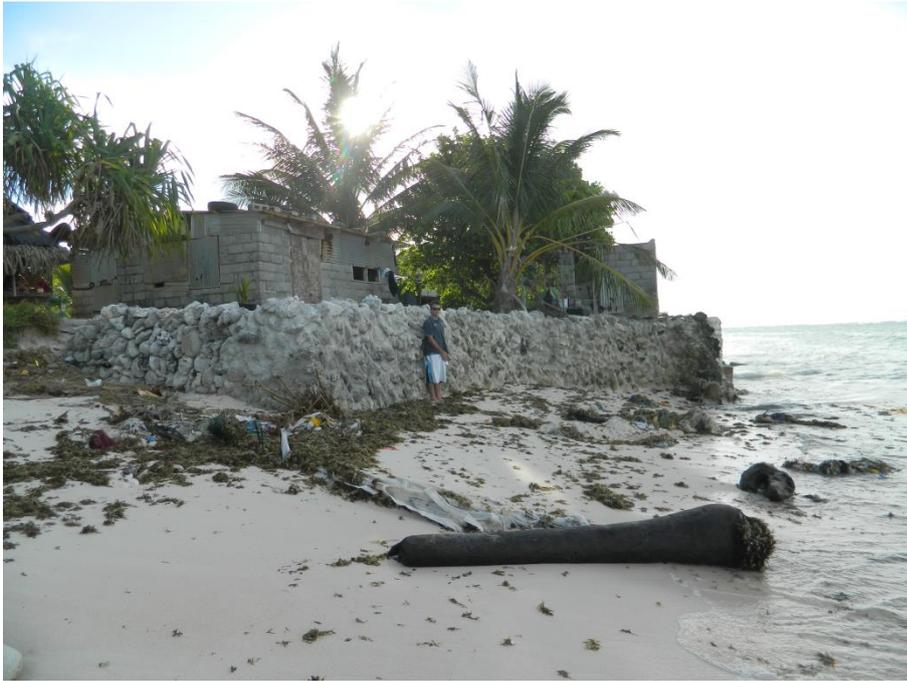
**Figure 23:** A seawall structure at Bonriki. Vertical hard structures such as these can lead to scour of the beach and interrupt longshore sediment transport, which can lead to erosion along the adjacent shoreline
