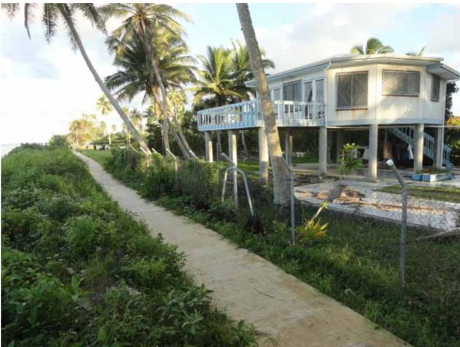
Figure 15: House in the backshore of Nuku'alofa built using a concrete stilt construction. Even though the house is elevated to mitigate against flooding and wave action during storm events, it is located in a vulnerable area close to the shoreline.
