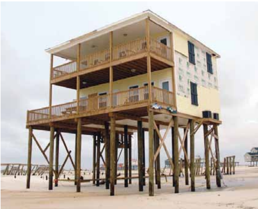
Figure 13: A successful, well-elevated and embedded pile-foundation building.
