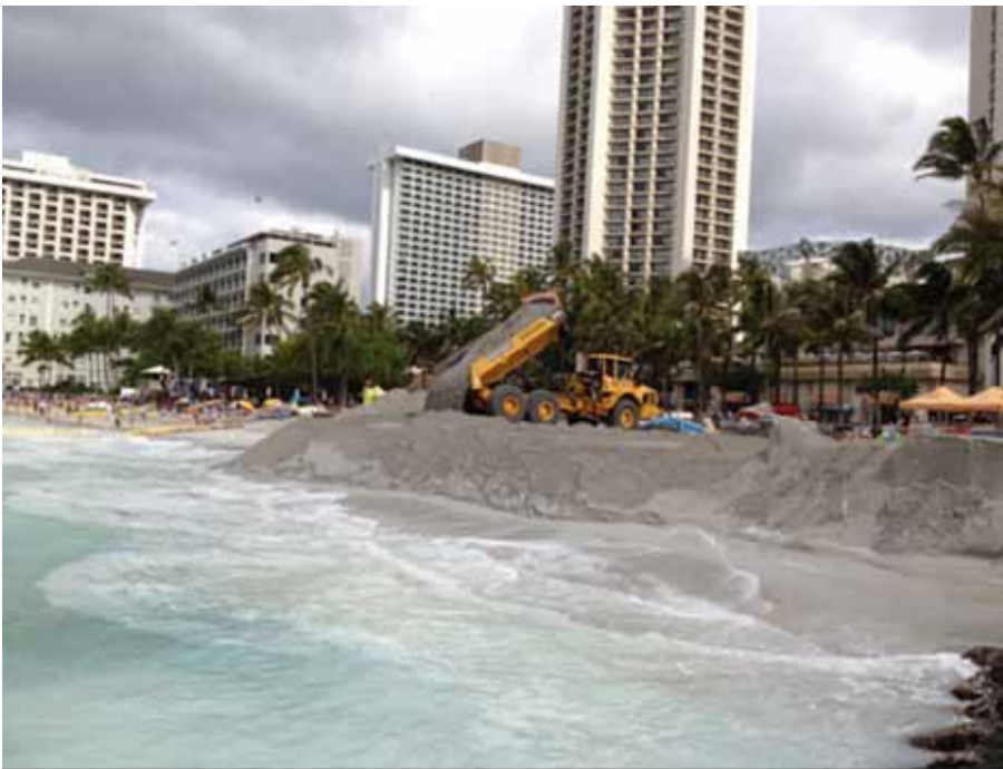
Figure 5: Beach recharge work in progress
