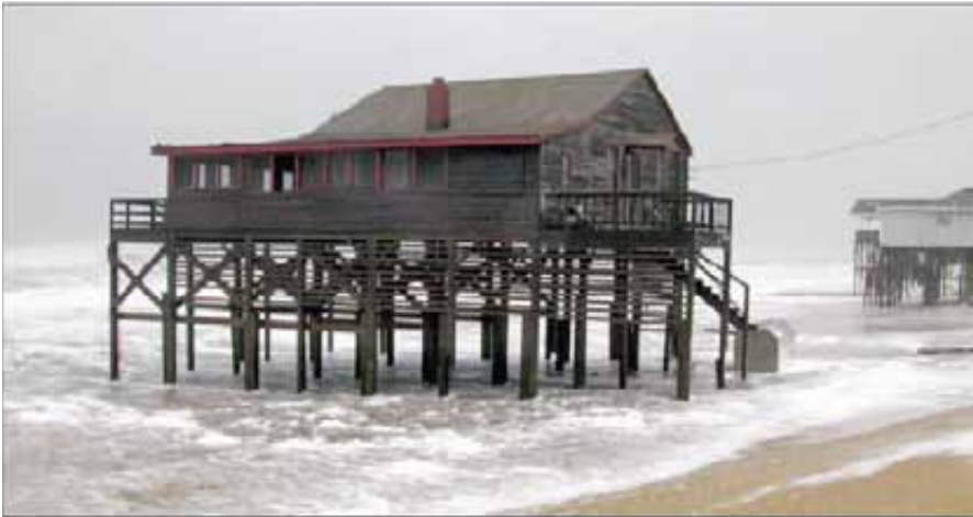
Figure 14: Sound coastal buildings rendered uninhabitable by erosion
