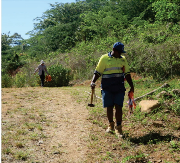
Figure A4.5.1. Setting up a survey profile using a measuring tape to guide the laying of electrical cables.
