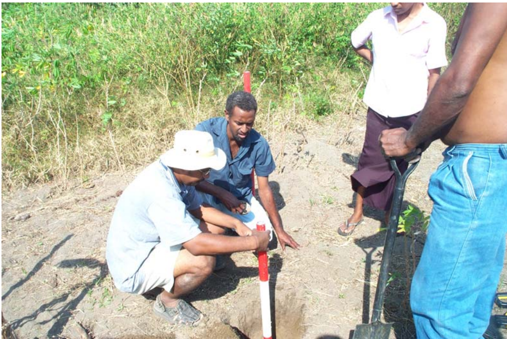
Installation of the Permanent Ground Control Survey Mark for the Beach Profile Survey in Mele Bay.
