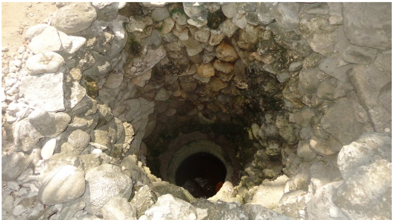
Figure A11-2. Well using both concrete rings and coral rocks as casing materials.
