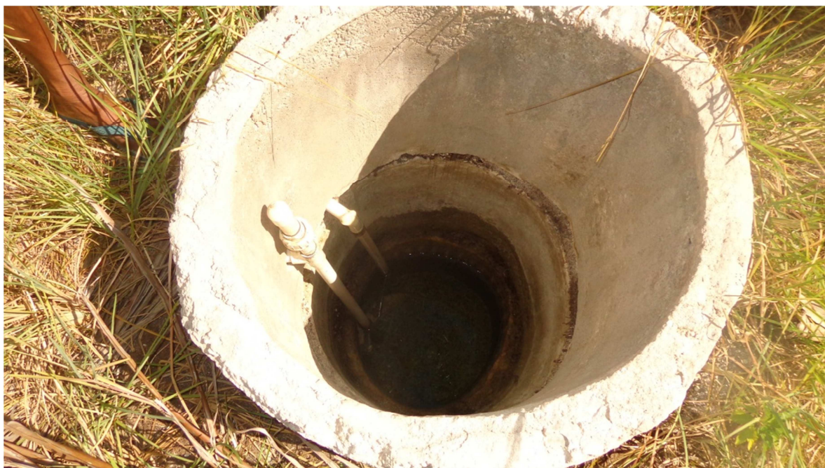
Figure A11-3. Multiple Tamana pump distribution lines from a communal well.
