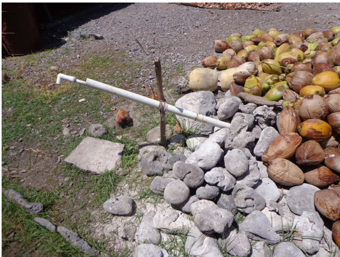
Figure 11. A Tamana pump connected to a completely covered well in Aoniman Village.
