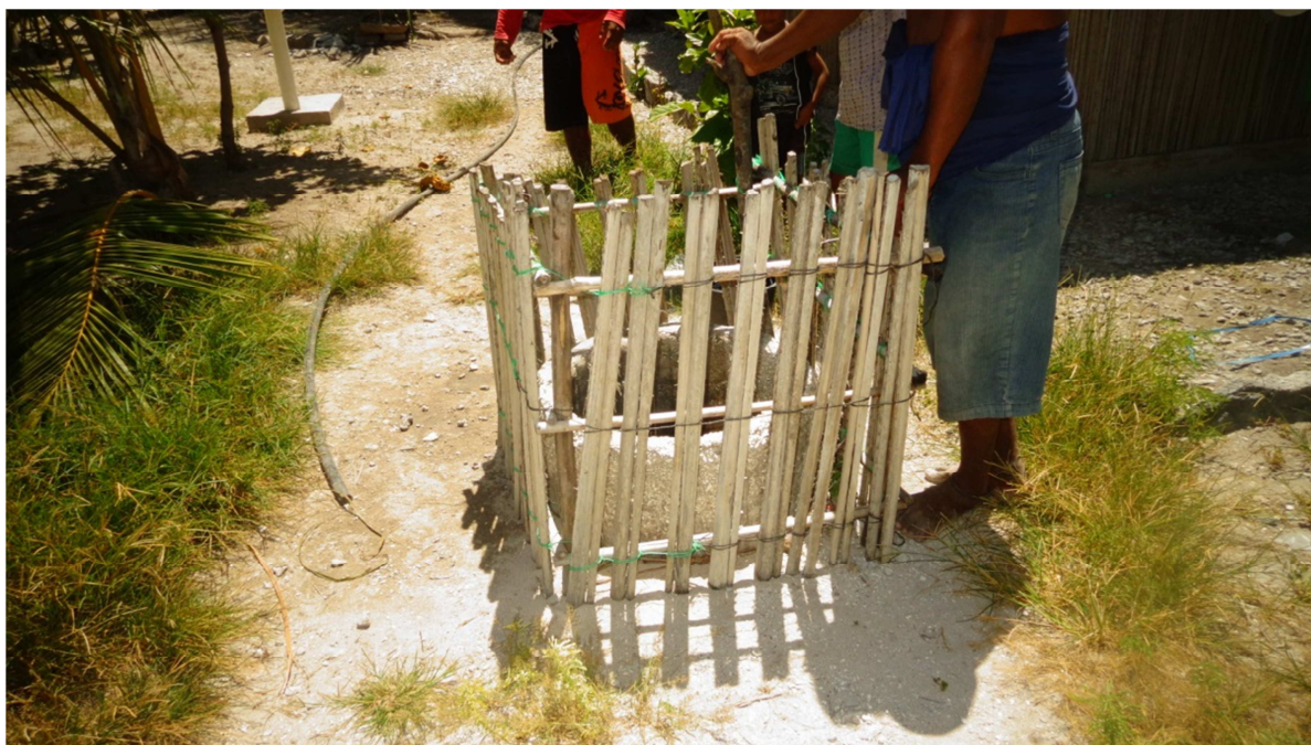
Figure A11-7. Example of timber fencing to regulate access to wells.
