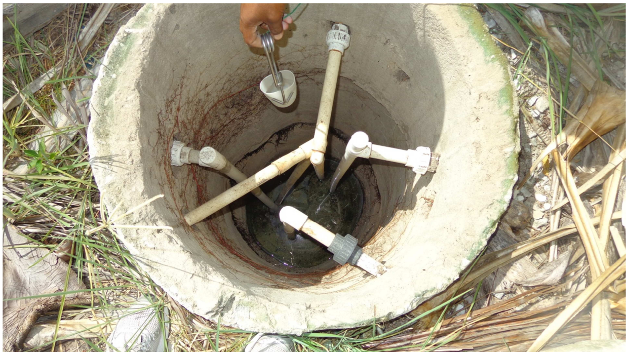
Figure 10. Multiple Tamana pumps installed in a communal well for Taubukiniberu Village.
