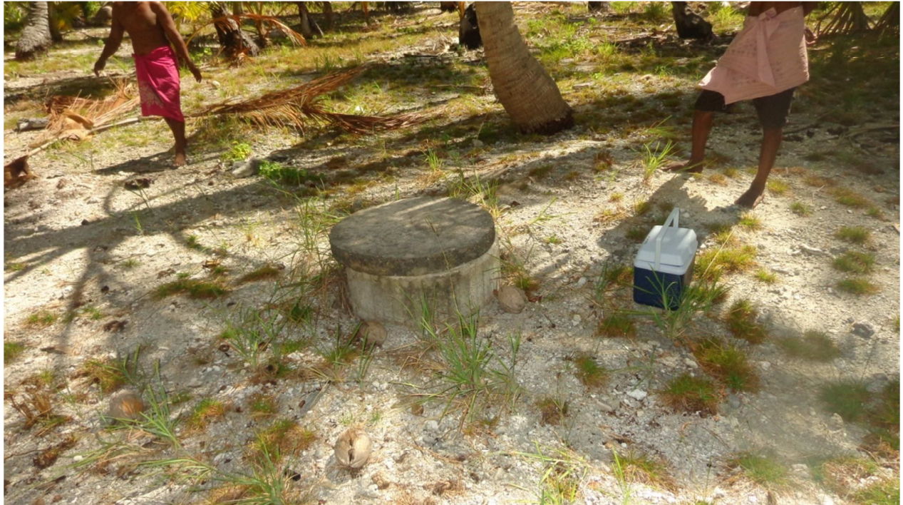
Figure A11-1. A covered communal well, abstracted by hand pump, Autukia Village.
