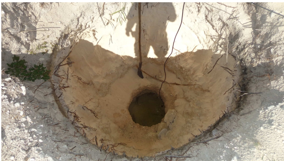
Figure A11-4. Example of an uncased well in Autukia Village.
