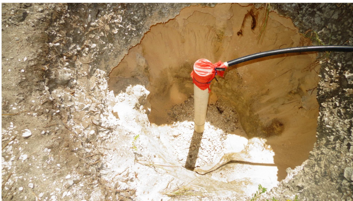
Figure A11-6. A partially buried well accessed by Tamana pump and using PVC pipe
