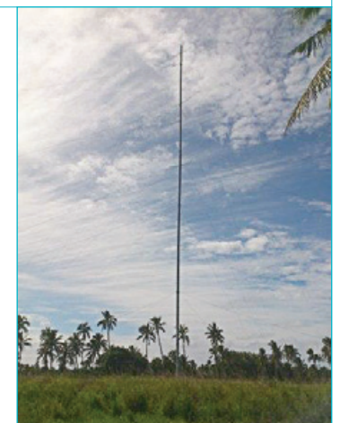
50m tall wind monitoring mast at Lapaha in Tongatapu, Tonga Photo by: SPC/GIZ CCCPIR
