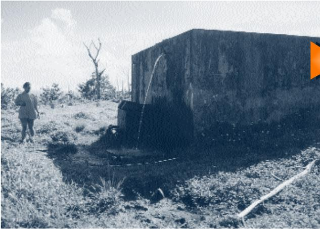
A river surface water collecting system: the water sits in the holding tanks before being redistributed to villages. The water in the tanks is not treated, even though analyses have shown that river surface water may be contaminated by faecal germs.
