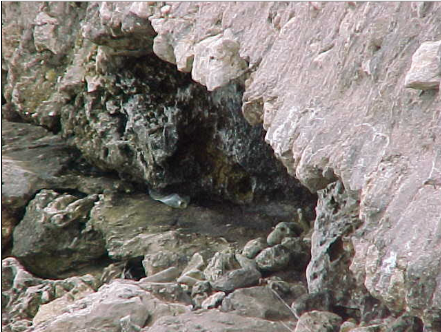
Figure 21. Removal of boulder aggregate at the base of the retaining wall on the eastern side of the structure.
