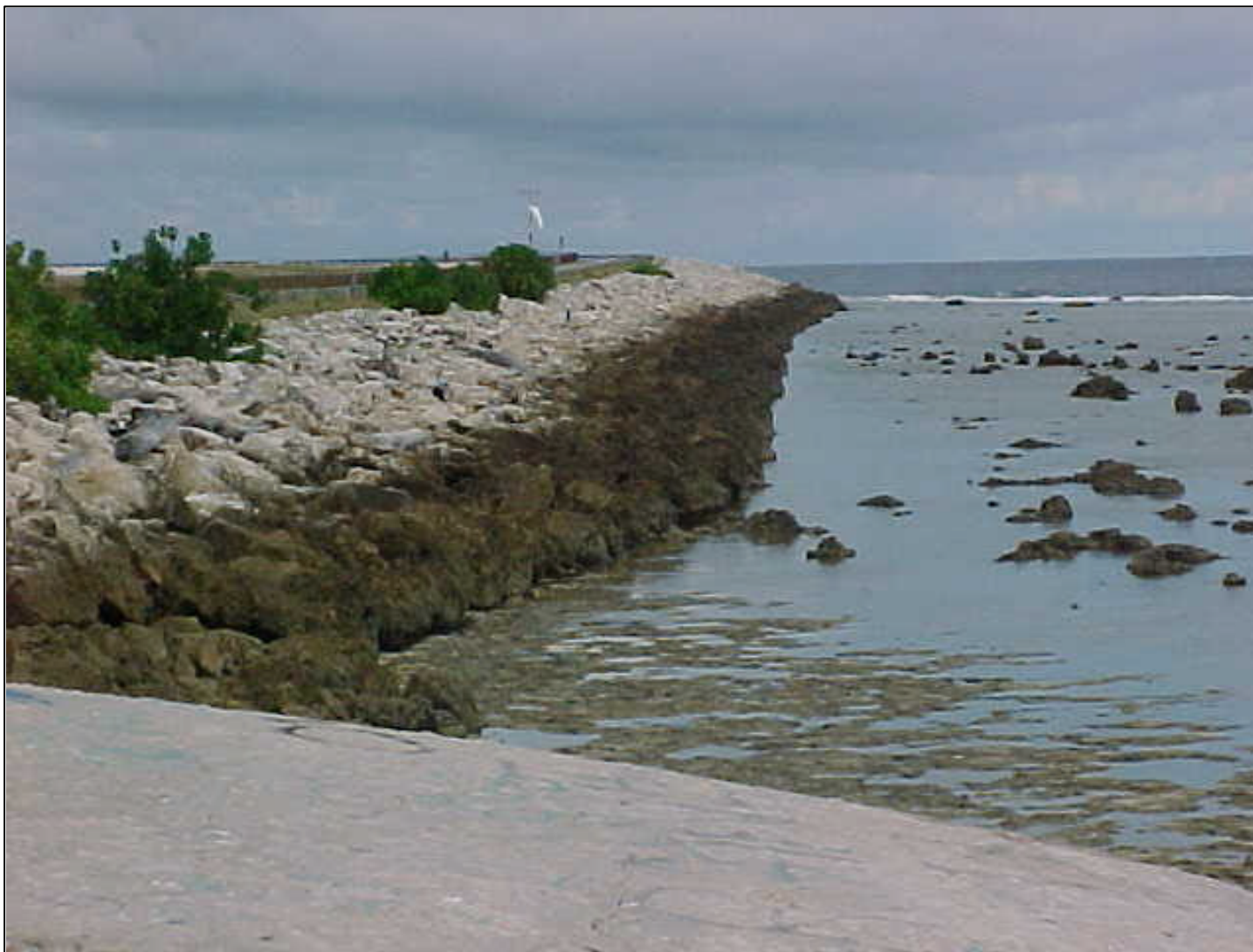
Figure 15. Details of the limestone rip-rap revetment along the airport fill site.
