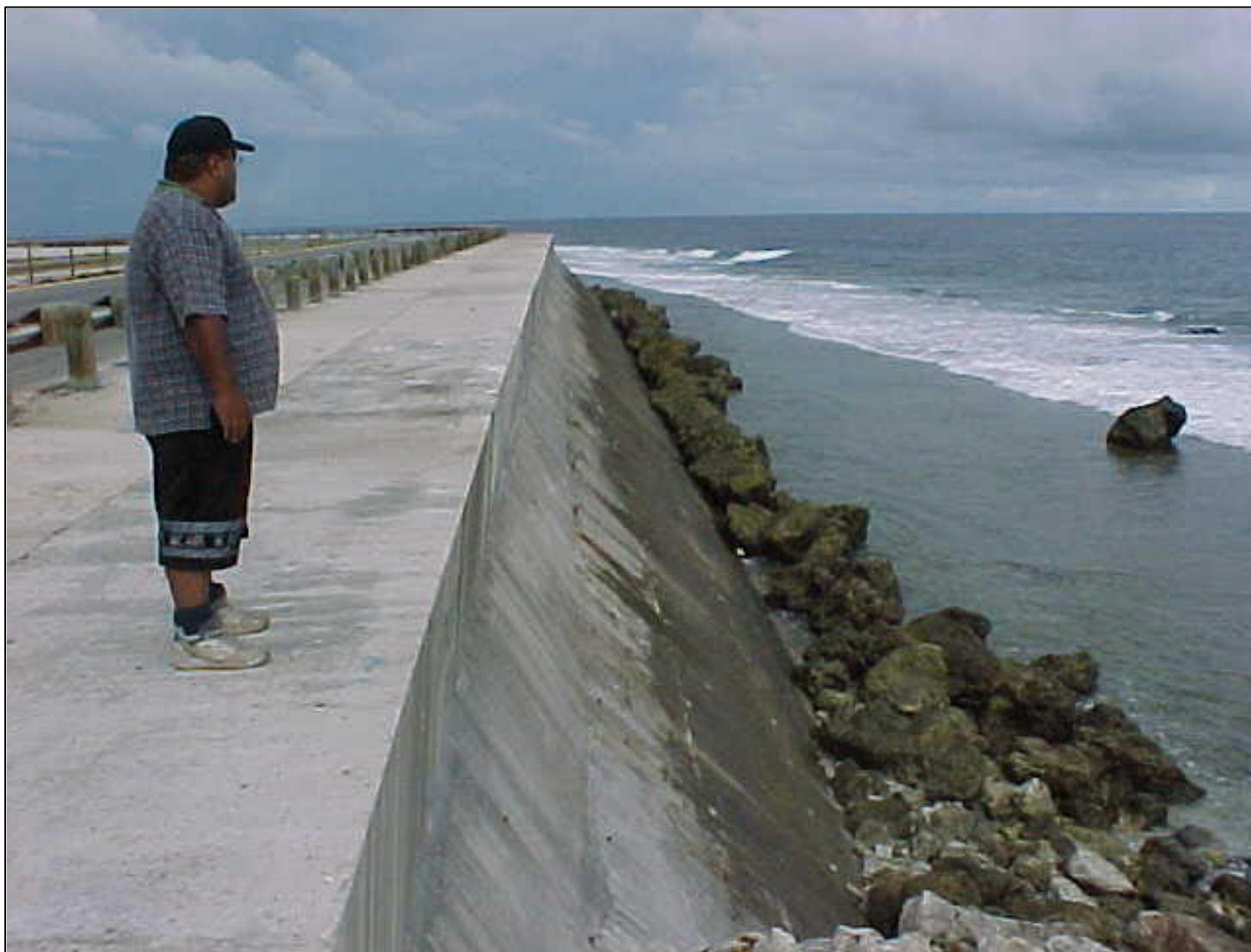
Figure 26. Gravity concrete retaining wall at the outer perimeter of the airport fill site. Looking east.
