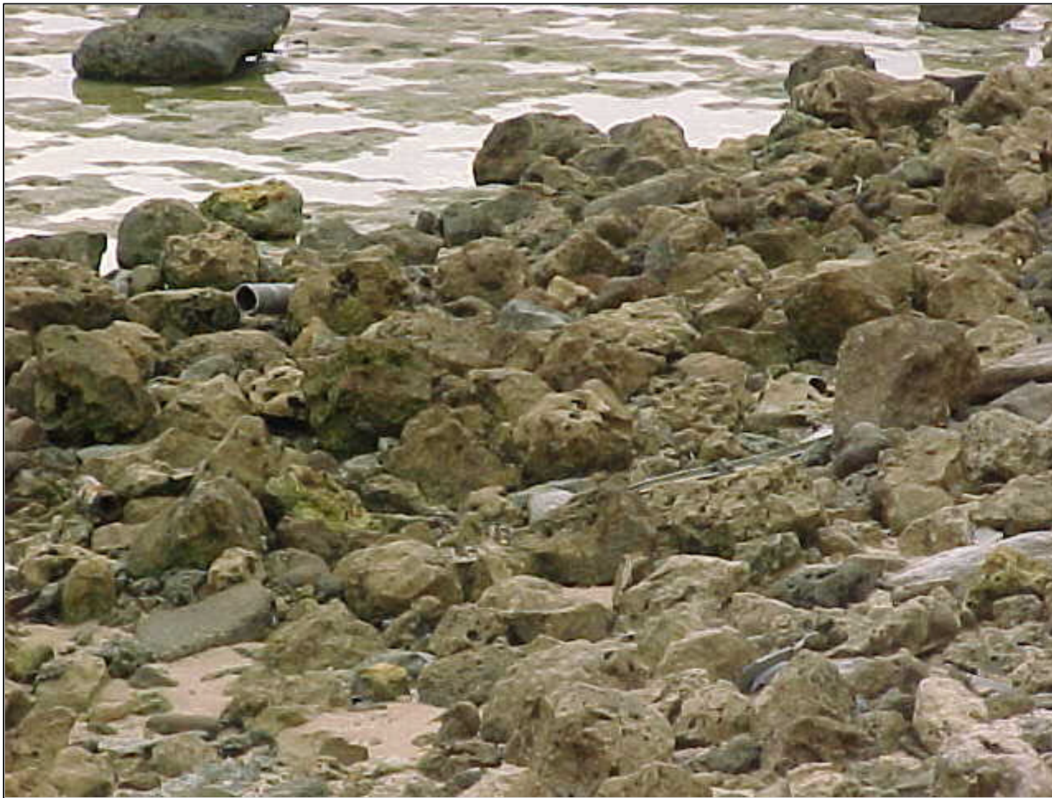
Figure 17. Limestone boulders from failed coastal protection structures.
