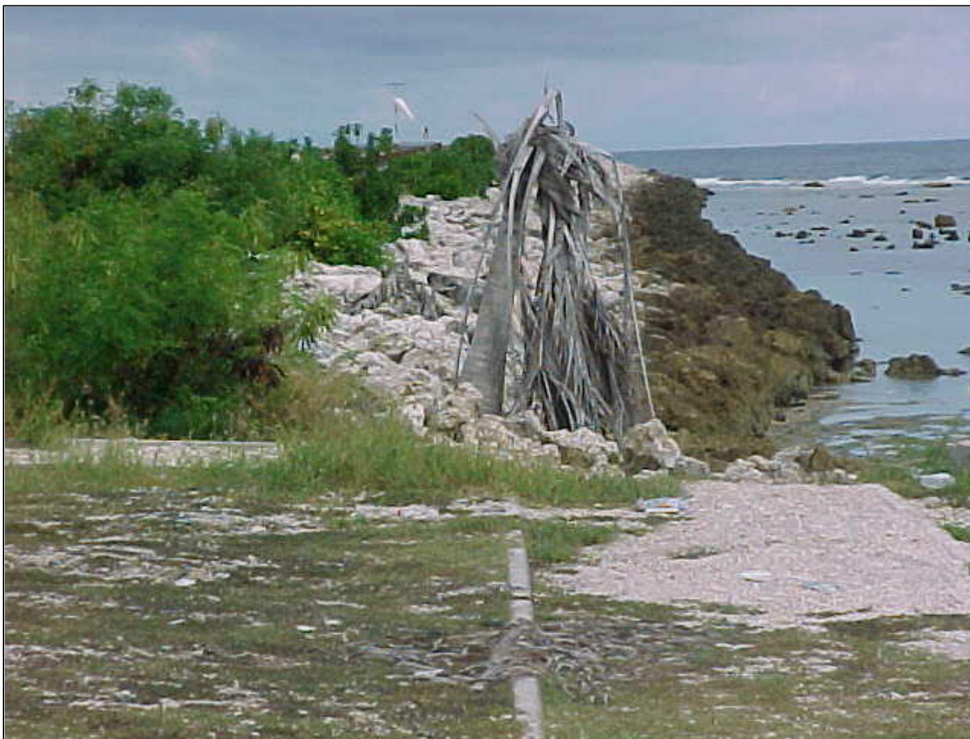
Figure 14. Details of the fill protection using rip-rap revetment.
