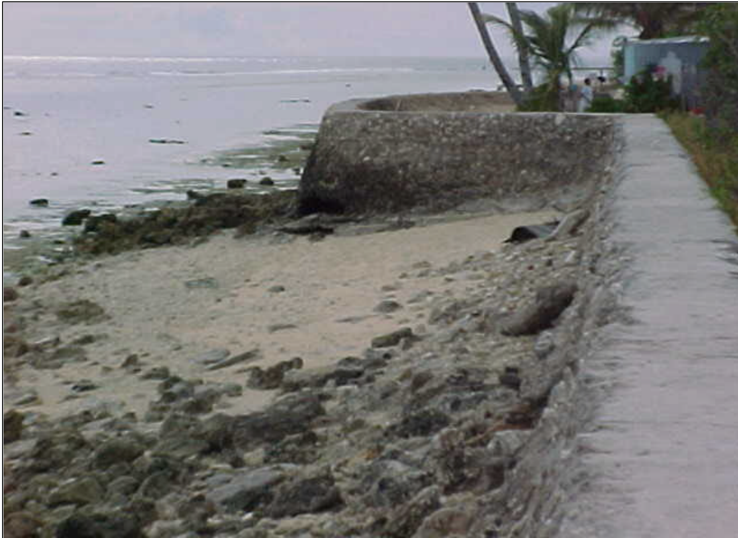
Figure 16. Part of an old masonry retaining wall at the erosion site.
