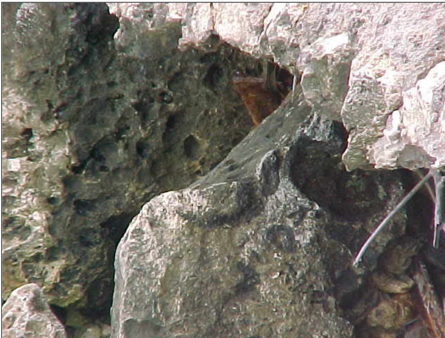
Figure 20. Large cavities at the base of the scoured retaining wall.
