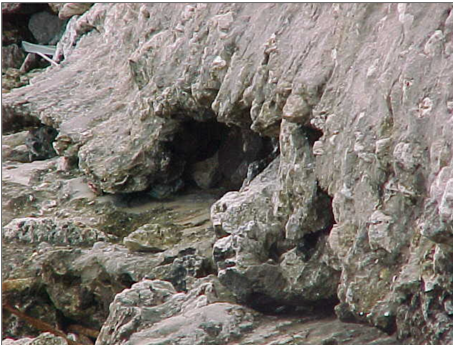
Figure 22. Scouring and removal of wall aggregate due to wave action and abrasion.
