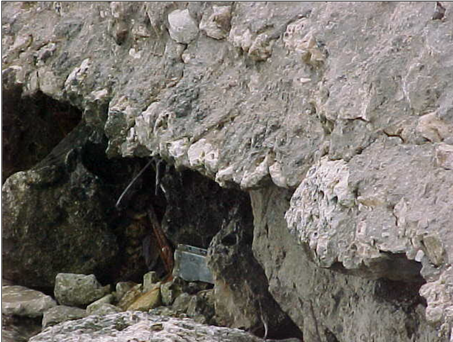
Figure 19. Details of the scoured western section of the scoured retaining wall.
