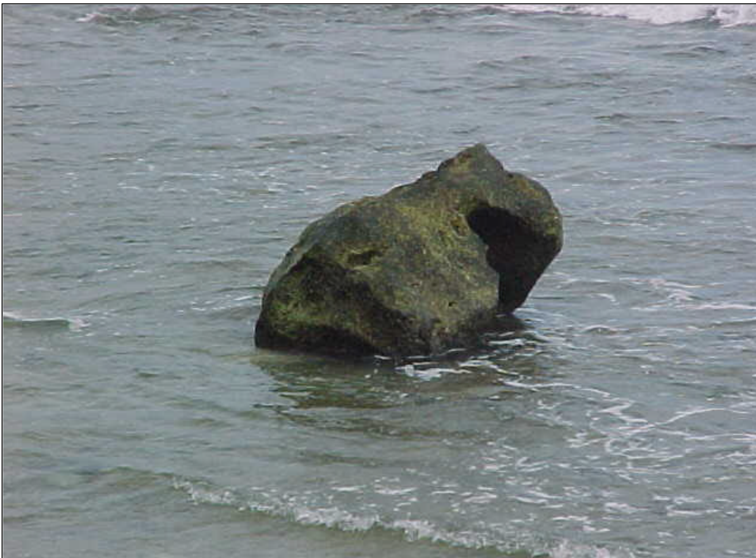
Figure 27. Dislodged limestone rip-rap boulder removed from the base of the gravity wall (Figure 26).
