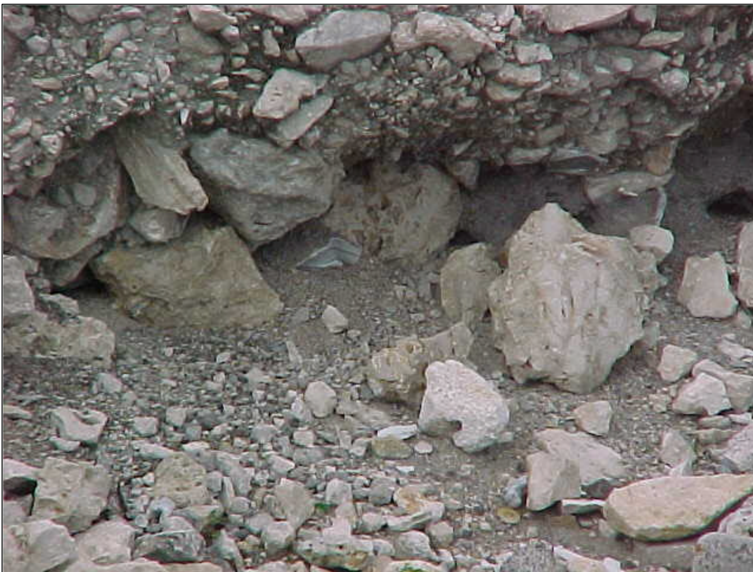
Figure 25. Characteristics of the scoured area at the erosion scarp in Figures 23 and 24. Note the exposed aggregate fill.
