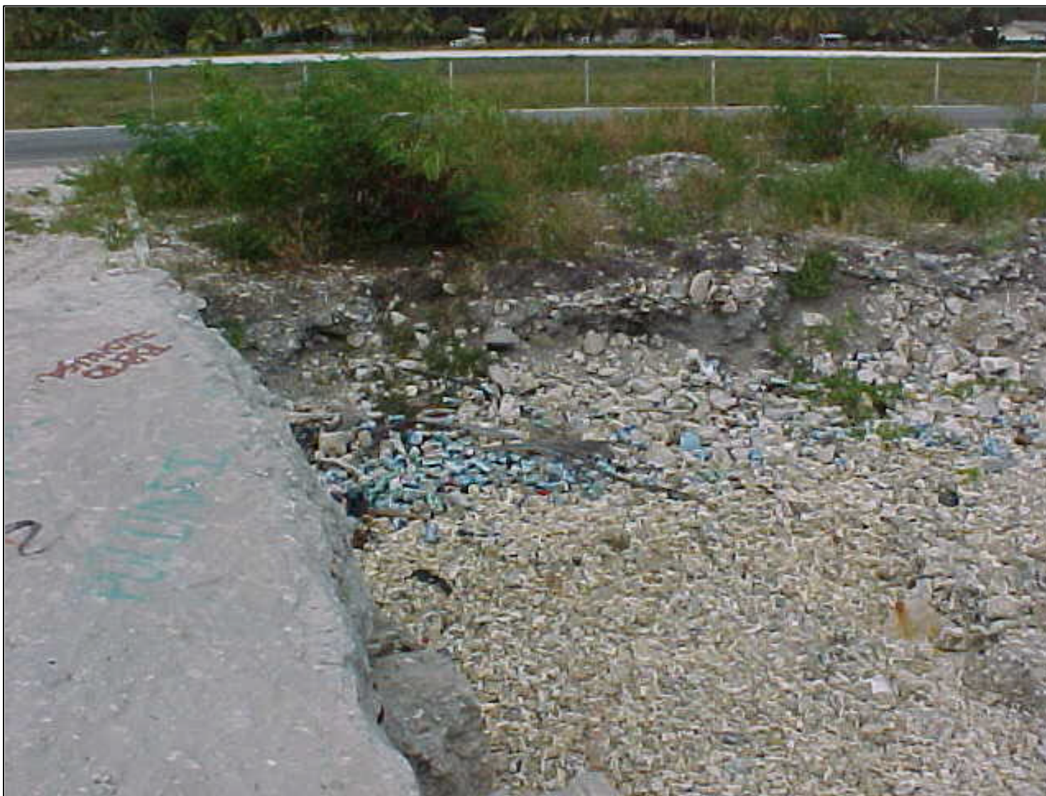
Figure 23. Erosion scarp at the western end of the airport rip-rap revetment.
