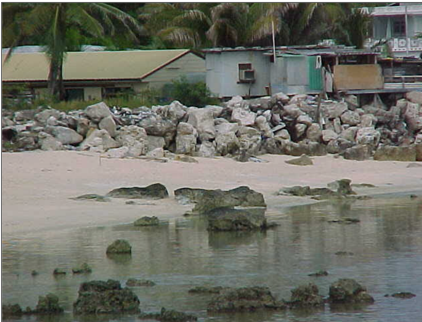
Figure 32. View looking northeast, showing randomly placed limestone boulders for protection of residential property along the natural coastline to the East of the airport fill site. Note the gentle sandy beach and natural limestone pinnacle in the water.
