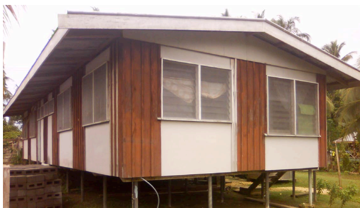
Example of a Solomon Island house built on galvanised steel pipes
