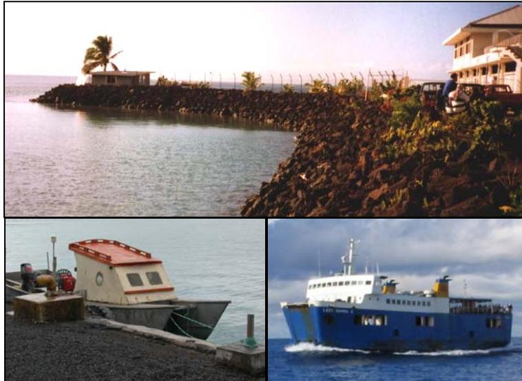
Fig. 23. The seawall at the Salelologa wharf in 1998 (upper); the newly-built Salelologa wharf (lower left) at which a big car ferry, the lady Samoa II (lower right), could berth. Note the well-constructed concrete wall beside a small boat. Lower pictures were taken in 2005.
