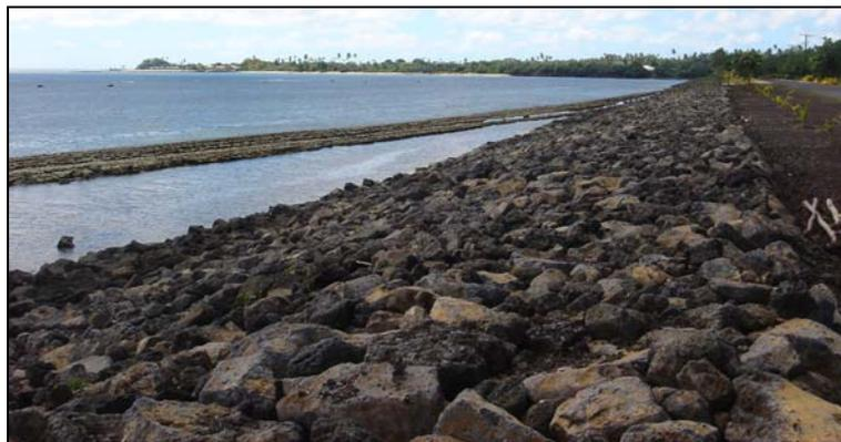
Fig. 24. A seawall made of gravels and boulders without cementation.
