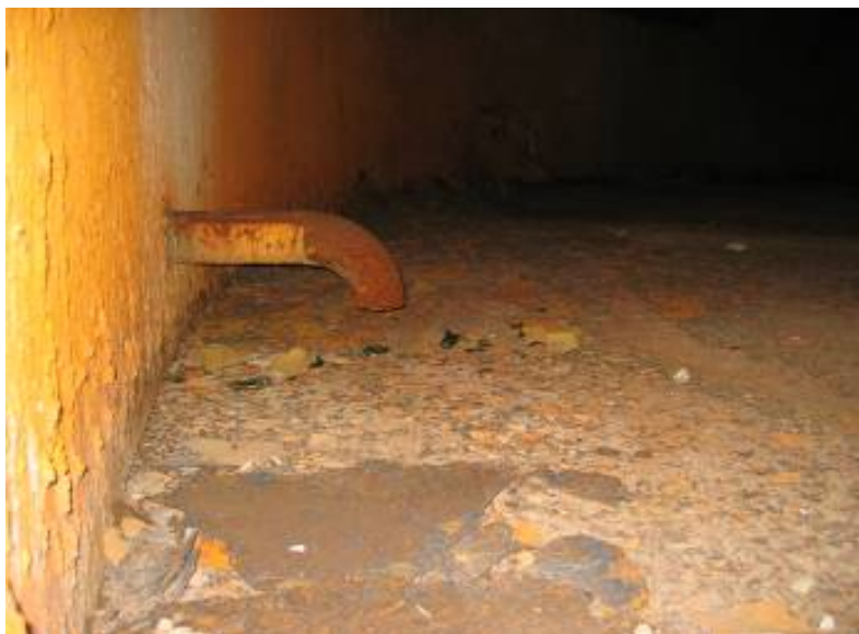
Corrosion of Decommissioned Water Storage Tank Floor.
