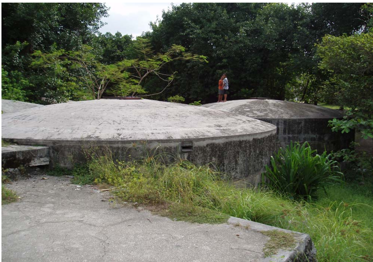
Nauru – Reinforced concrete water storage tanks (derelict)
