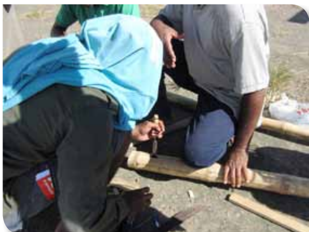
Figure 27. Cutting a slot for an end peg in the bamboo beam.
