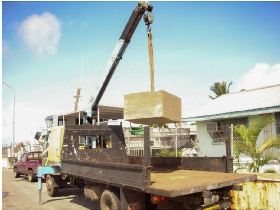
**Image 2.** Large cement block anchor being lifted by crane for deployment.
