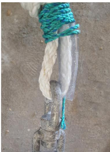
Image 1 shows a FAD that was poorly constructed. The FAD was in the water for less than one month before washing ashore. While the FAD was lost due to a different connection than the one pictured here, you can see that the whipping around the plastic tubing was not tight or long enough to hold the tubing in place. If other sections of this FAD did not break, eventually the tube would have cut the rope at this point.
