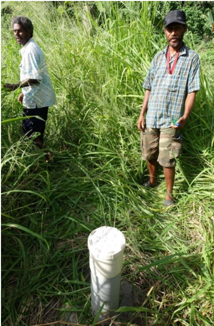
Figure 9. Borehole drilled by a private contractor along the coast. Several boreholes exhibited strong tidal influence in water level and quality.
