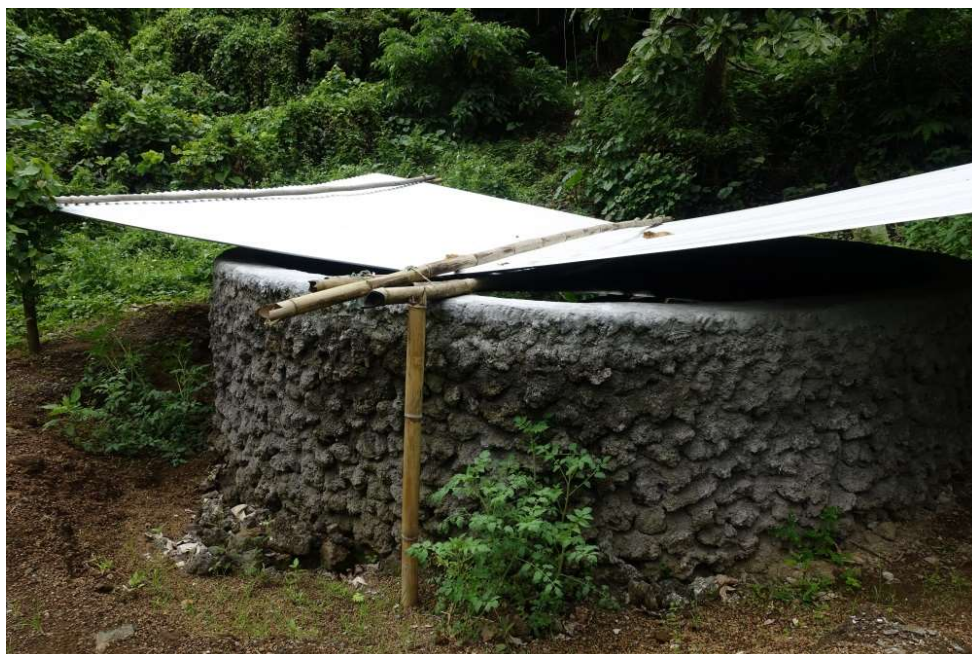
Figure 8. Privately owned catchment system comprising a constructed well raised above ground and two sheets of roofing iron inclined towards the centre of the well.
