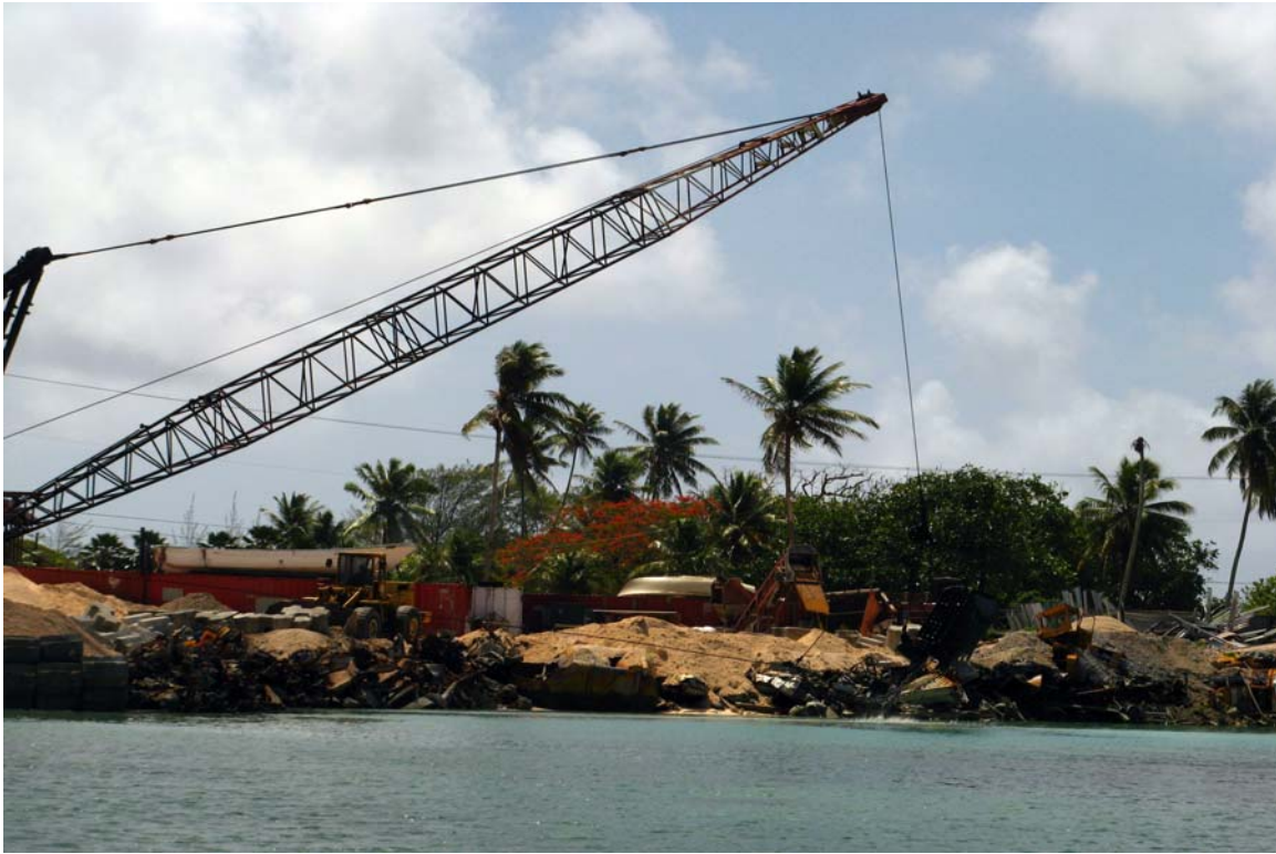
Figure 4. Shoreline based dragline scraper and crane system extracting sand and gravel from the Majuro Lagoon.
