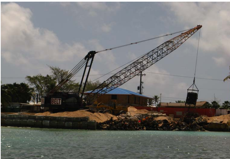
Figure 23. Photo of the present shore based dredging operation at Site DL.
