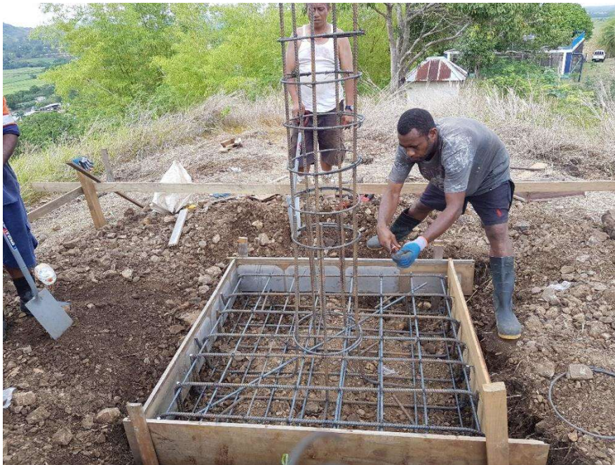
Figure 6: Construction of the GNSS CORS Pillar
