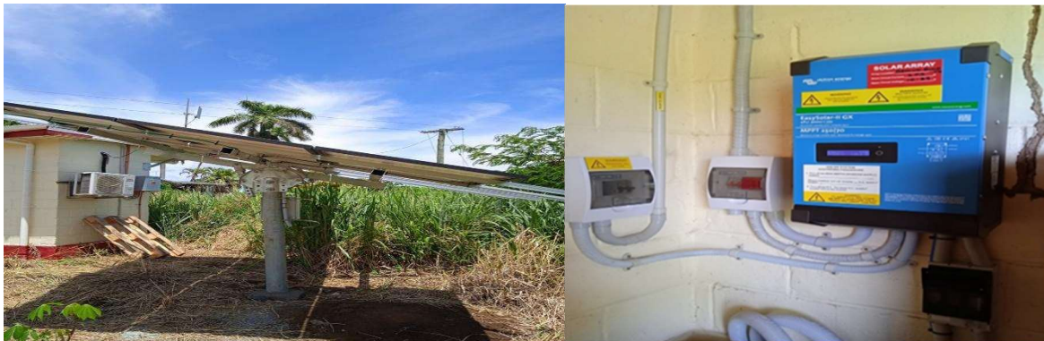
Figure 13: Typical solar power set-up at the GNSS CORS Site in Ono-i-lau, Lakeba and Koro
