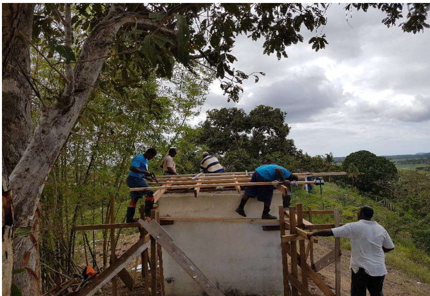
Figure 7: Construction of the GNSS CORS hut
